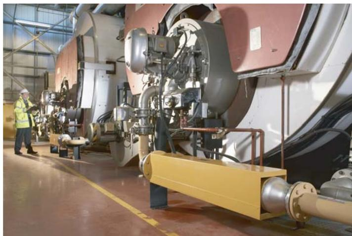
*"The installation was carried out by Maxsys Fuel Systems Ltd during our Christmas shutdown. In mid March 2005 we received a report from ABB showing a 5% reduction in gas consumption per tonne of steam produced... during a 20 day period 12,400m<sup>3</sup> less gas was consumed than would have been expected if the Fuel System had not been installed. I was so pleased with the results that we asked Maxsys to install a further Fuel System on to another boiler". Mike Fisher, General Manager.*
