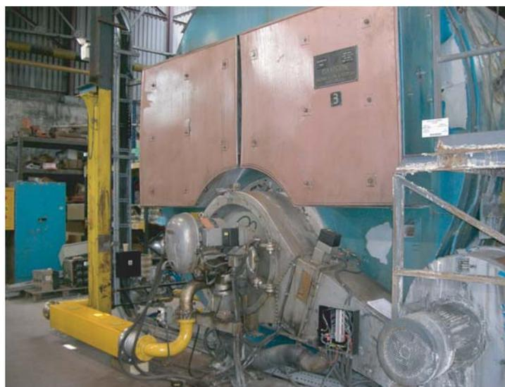
This heavy steam demand is provided by one central boiler house which raises around 20 to 25 tonnes of steam per hour.
